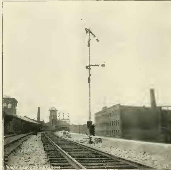
INTERLOCKING ELECTRIC SLOT "HOME" SIGNAL AT NEWARK, N. J.—D. L. & W. MARKED B IN DIAGRAM.
